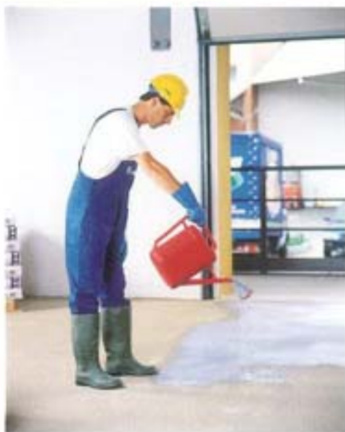
Applying PRIMER G to improve adhesion before leveling with PLANO 3
