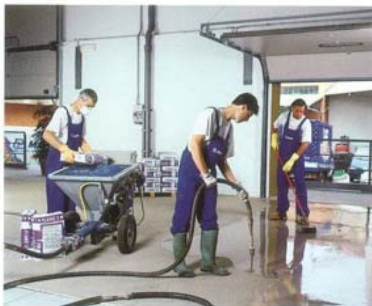
Applying PLANO 3 self-leveling smoothing compound with a pump
