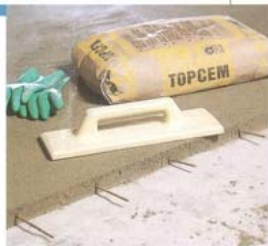
Detail of TOPCEM screed with reinforcing
