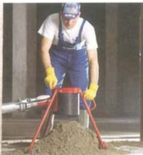
TOPCEM mix being applied with a pump
