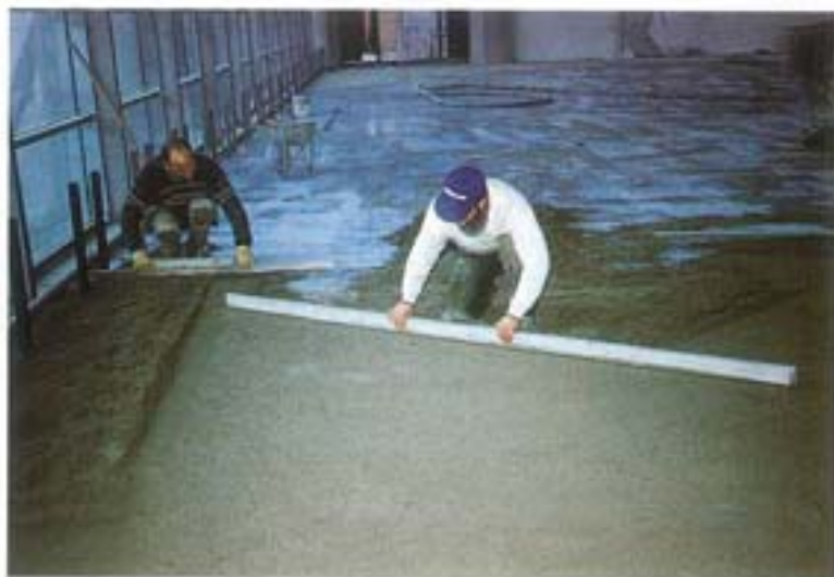
Portello convention center, Milan, Italy. TOPCEM screed
