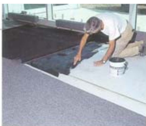
At left, Hewlett-Packard offices, Slezzano, Italy. ADESILEX G19 CONDUCTIVE tests used to install pvc flooring At right: conductive cementitious adhesive used to install conductive ceramic tiles
