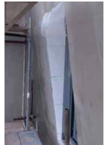
LEFT. An external view of the new Tryp Lisboa Aeroporto Hotel in Lisbon. ABOVE. Application of the MAPETHERM insulating system on the hotel's external façades.
