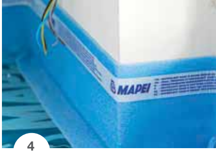
PHOTO 1. The MAPESILENT ROLL sheets were laid over the concrete surface with the fibre side facing down. PHOTO 2. The sheets were overlapped by 5 cm to prevent the formation of acoustic bridges. PHOTO 3. After making sure the various sheets of MAPESILENT ROLL were perfectly positioned, MAPESILENT BAND R 50/160 was applied around the perimeter of walls and all the overlaps were sealed with MAPESILENT TAPE. PHOTO 4. MAPESILENT BAND R 50/160 adhesive membrane was placed along the walls.
