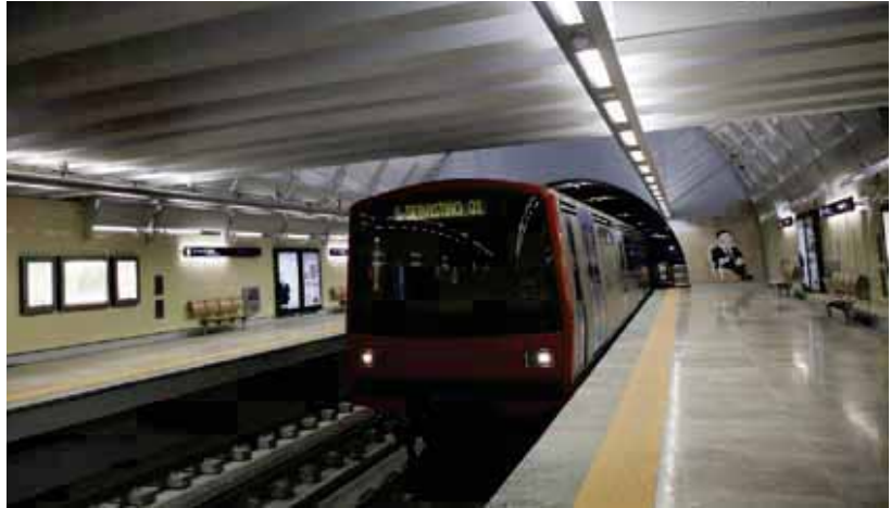
ABOVE. The porcelain tiles for the platforms were bonded with KERALASTIC T and joints were grouted with ULTRACOLOR PLUS.
