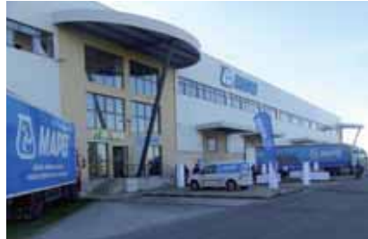
LEFT. The Lusomapei headquarters in Castanheira do Ribatejo in central Portugal.
