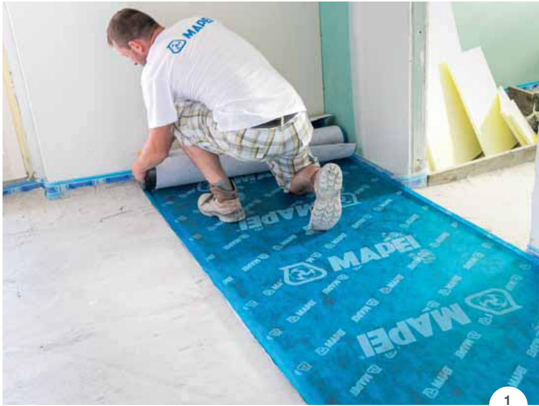
PHOTO 1. The MAPESILENT ROLL sheets were laid over the concrete surface with the fibre side facing down. PHOTO 2. The sheets were overlapped by 5 cm to prevent the formation of acoustic bridges. PHOTO 3. After making sure the various sheets of MAPESILENT ROLL were perfectly positioned, MAPESILENT BAND R 50/160 was applied around the perimeter of walls and all the overlaps were sealed with MAPESILENT TAPE. PHOTO 4. MAPESILENT BAND R 50/160 adhesive membrane was placed along the walls.
