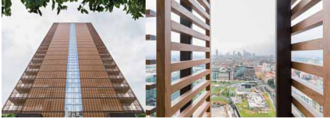
An image of the Giax Tower. The building has electrically-operated sun-shades with horizontal blades.
