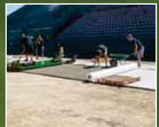
PREPARING AND APPLYING THE DRAINAGE MIX WITH Mapesoil VD
