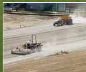
STABILIZING WITH Mapesoil 50
