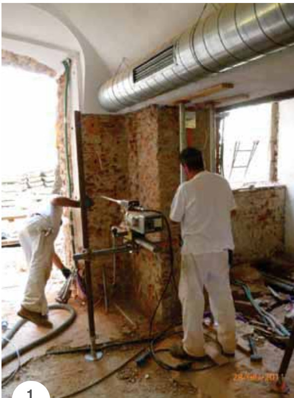
PHOTO 1. Horizontal holes for the steel bars.
