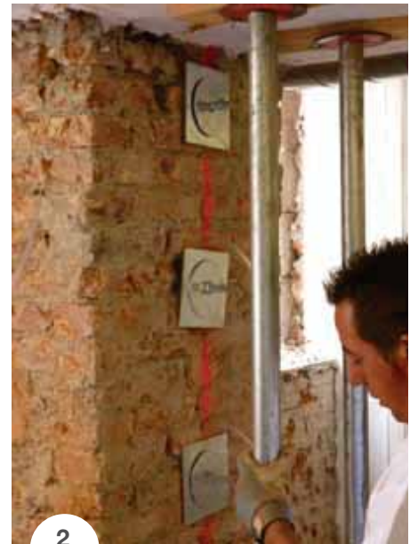
PHOTO 2. Positioning the plates.
