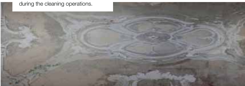
THE DUCHESS OF GENOA'S APARTMENT: a section of the vault during the cleaning operations.
