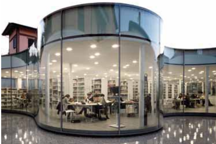
LEFT. The new city library in Maranello (Central Italy).
