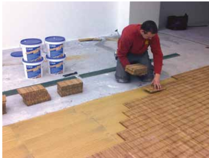
ABOVE. Before installing the wooden floor, the substrates were treated with PRIMER G. BELOW. After smoothing and levelling the substrate with MAPESOL 3, the wooden floor was bonded with ULTRABOND ECO S955 1K adhesive.
