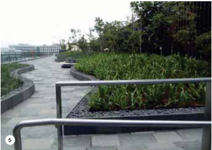
PHOTO 4. For external driveways (e.g. drop-off points), walkways and atrium, KERAFLEX MAXI S1 was used to bond granite slabs and joints were grouted with KERACOLOR GG.
