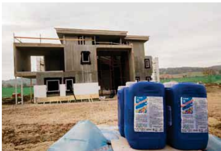
ABOVE. Before installing the covering on the façades using ELASTORAPID adhesive, the walls were thermally insulated with MAPETHERM TILE SYSTEM.
