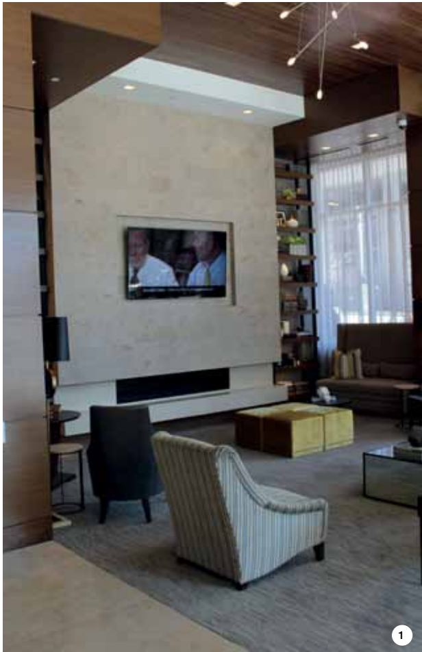
PHOTO 1. The installers cut the tile surrounding the fireplace down to 22,9 x 91 cm to create a beautiful floor-to-ceiling backdrop for the lobby. In these areas, they used ULTRAFLEX LFT for bonding ceramic tiles and ULTRACOLOR PLUS for grouting joints. PHOTO 2. ULTRABOND ECO 995 was used to install the wooden flooring in the fourth floor club room and community kitchen.
