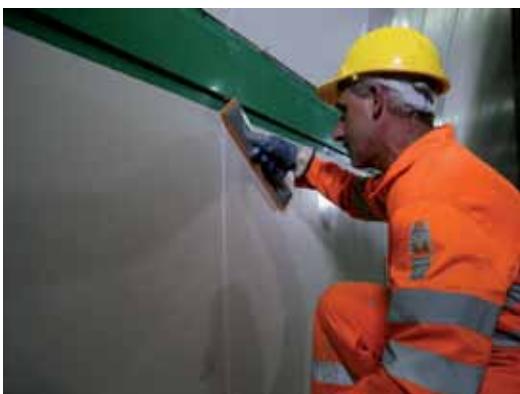
IN THESE PICTURES. Large-size ceramic tiles were bonded in the tunnel with KERAFLEX MAXI S1.
