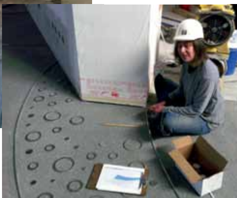
Some phases of the decoration of the floorings. The product chosen for the finishing was ULTRATOP PC.
