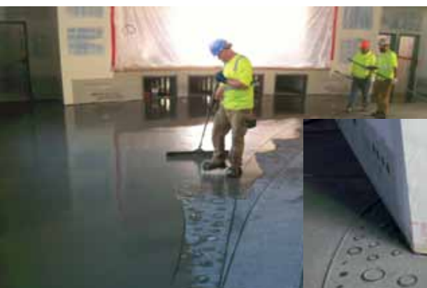
Some phases of the decoration of the floorings. The product chosen for the finishing was ULTRATOP PC.
