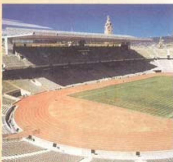
Athletic Stadium - Madrid Installation of rubber flooring using ADESILEX G19
