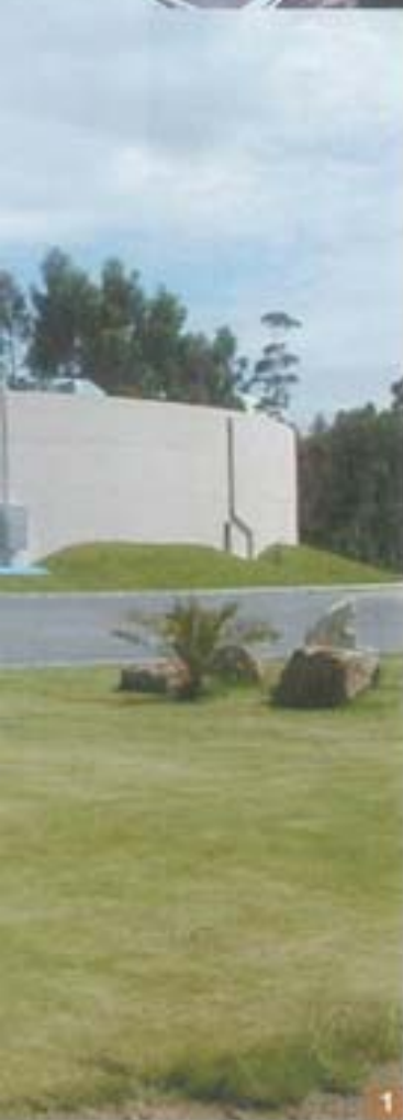
1. Exterior view of the tank with power supply and ventilation system
