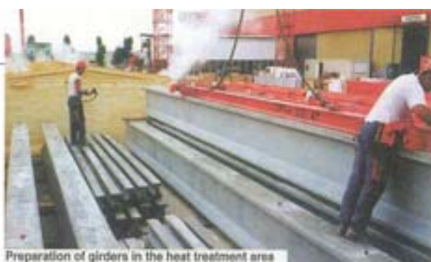
Preparation of girders in the heat treatment area
