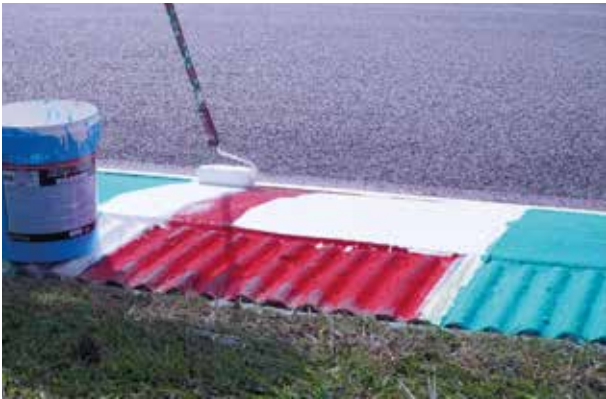
ABOVE. MAPECOAT TNS RACE TRACK was applied on the kerbs and run-off areas of the circuit.
