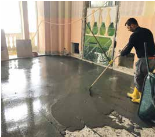
BELOW. PLANITOP HPC FLOOR 46 reinforced micro-concrete was used to strengthen the extrados of the floors of the Giuseppina Hall on the first floor.
