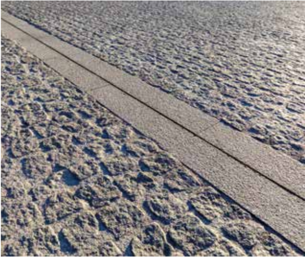
1 and 2. Application and cleaning of MAPESTONE PFS2 FLEX used to grout joints. 3. Samples of the mixes used to install (MAPESTONE TFB 60) and grout (MAPESTONE PFS2 FLEX) the stone paving were tested to make sure they were prepared correctly and complied with the specified performance properties. 4 The completed paving made up of stone slabs and cobblestones and the expansion joint.
