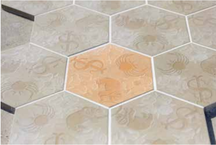
IN THIS PAGE. The porcelain tiles were installed along the promenades with KERAFLEX EXTRA S1 cementitious adhesive, with extended open time and no vertical slip.
