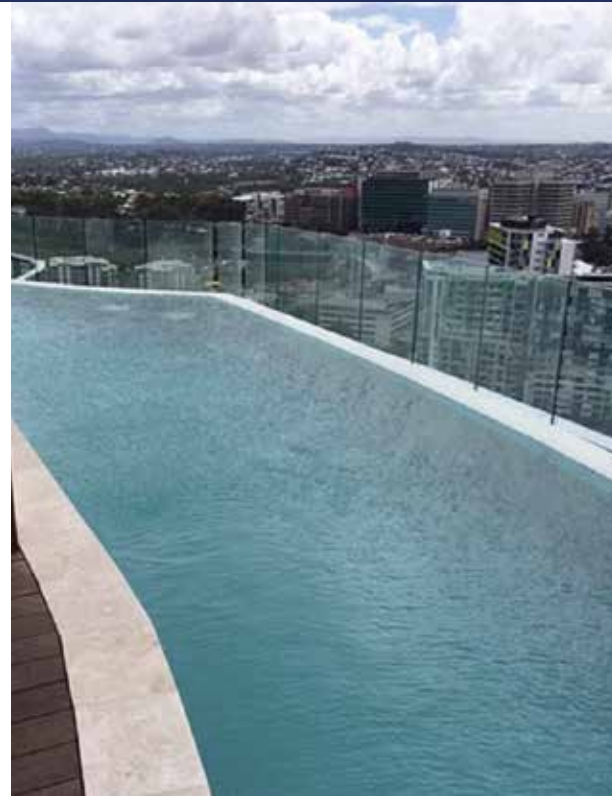
LEFT. KERAFLEX MAXI S1 was used to install ceramic and stone tiles on the walls and floors in numerous areas of the skyscraper. RIGHT. In the swimming pool on the 90 th floor, mosaic, tiles and stone slabs were bonded with KERABOND PLUS*+ISOLASTIC 50* and joints were grouted with KERAPOXY.
