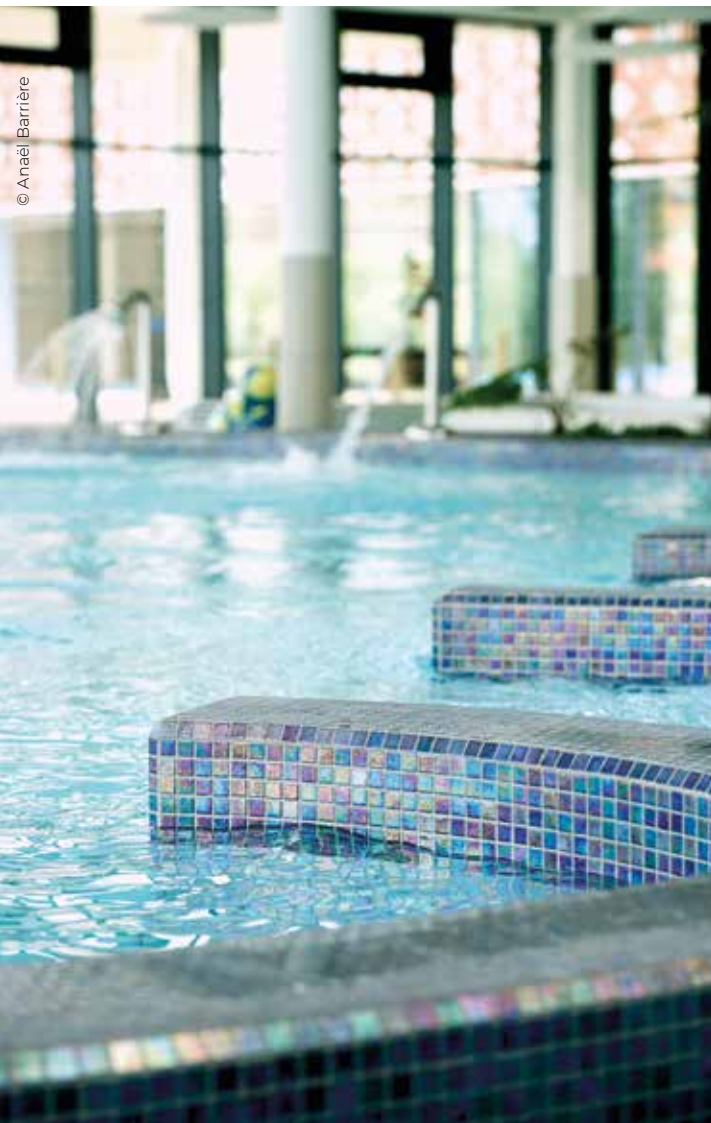
KERAPOXY CQ was used to install the mosaics in the pools and grout the joints.
