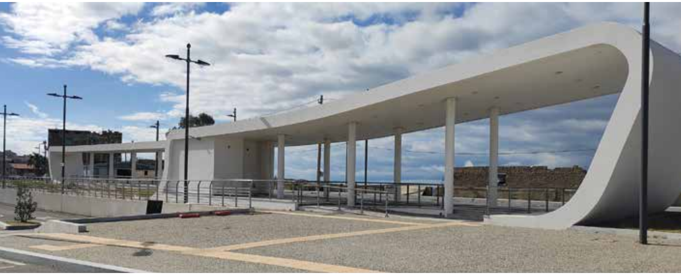
ABOVE. The surfaces of the shelter at the bus terminus in the port were waterproofed with MAPELASTIC flexible, two-component cementitious mortar.
