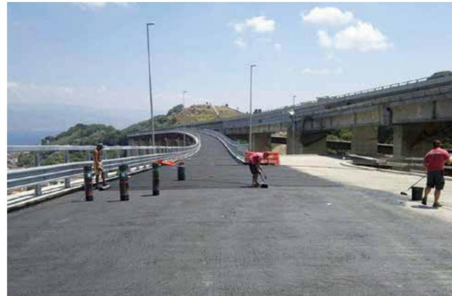
Preparing the installation layer with a primer for bituminous membranes. Using bituminous membranes on road surfaces allows to increase the durability and resistance of road surfaces, reducing maintenance costs.
