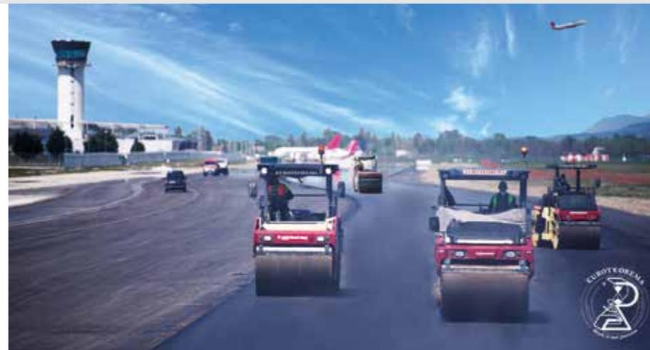
**LEFT.** Spreading and compacting the wear layer for the taxiways made up of bitumen modified with MAPEI E-SBC 2.
