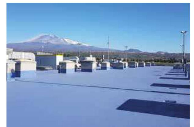
PURTOP 1000 polyurea membrane was chosen to waterproof the substrates of the carpark on the roof. It was applied by spray using a high-pressure bi-mixer pump.
