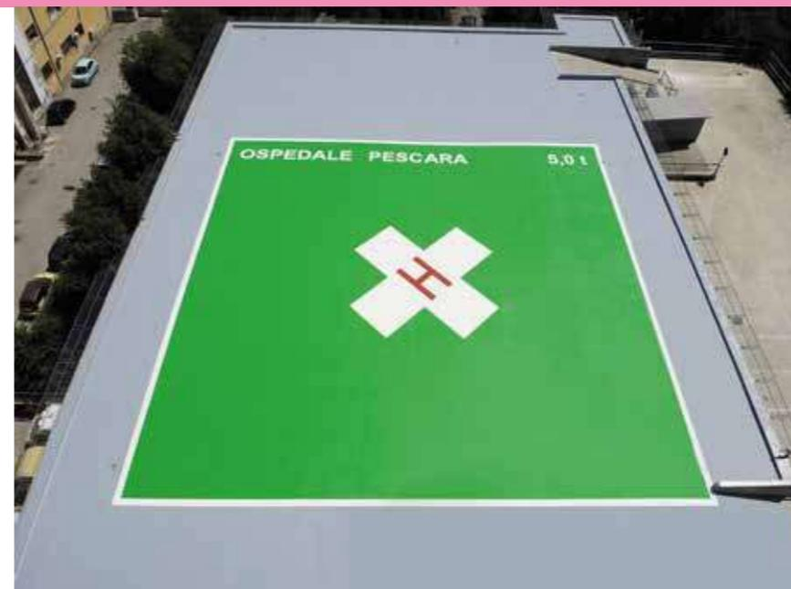
After treating the substrates with PRIMER SN+QUARTZ 0.5 and, in some areas, with PRIMER EP RUSTOP, surfaces were waterproofed with PURTOP 1000 polyurea membrane. Surfaces were then finished with MAPECOAT TC coloured, wear-resistant, aliphatic polyurethane finish.
