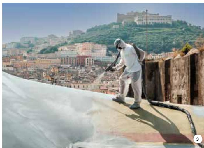
and a thickness of around 2 mm. This system adheres firmly to substrates and, after reticulation, forms a strong, continuous, and flexible membrane ready for foot traffic very soon after application. Thanks to its high tensile strength and crack-bridging capacity (including at low temperatures), this product is able to adapt to substrates of any shape or form without cracking.
