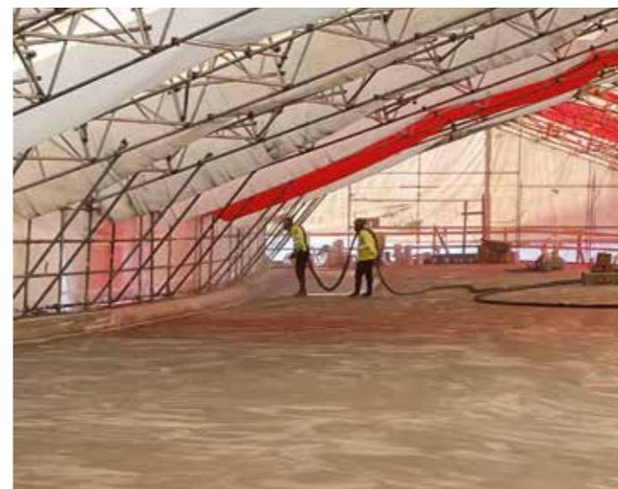
**ABOVE.** Hakaniemensilta Bridge is just a part of the prestigious Crown Bridges project which includes the construction of 3 bridges in the area to the east of Helsinki and the reconstruction of two existing bridges. Above, application by spray of PURTOP 400 M on several sections of the deck of the Hakaniemensilta Bridge.
