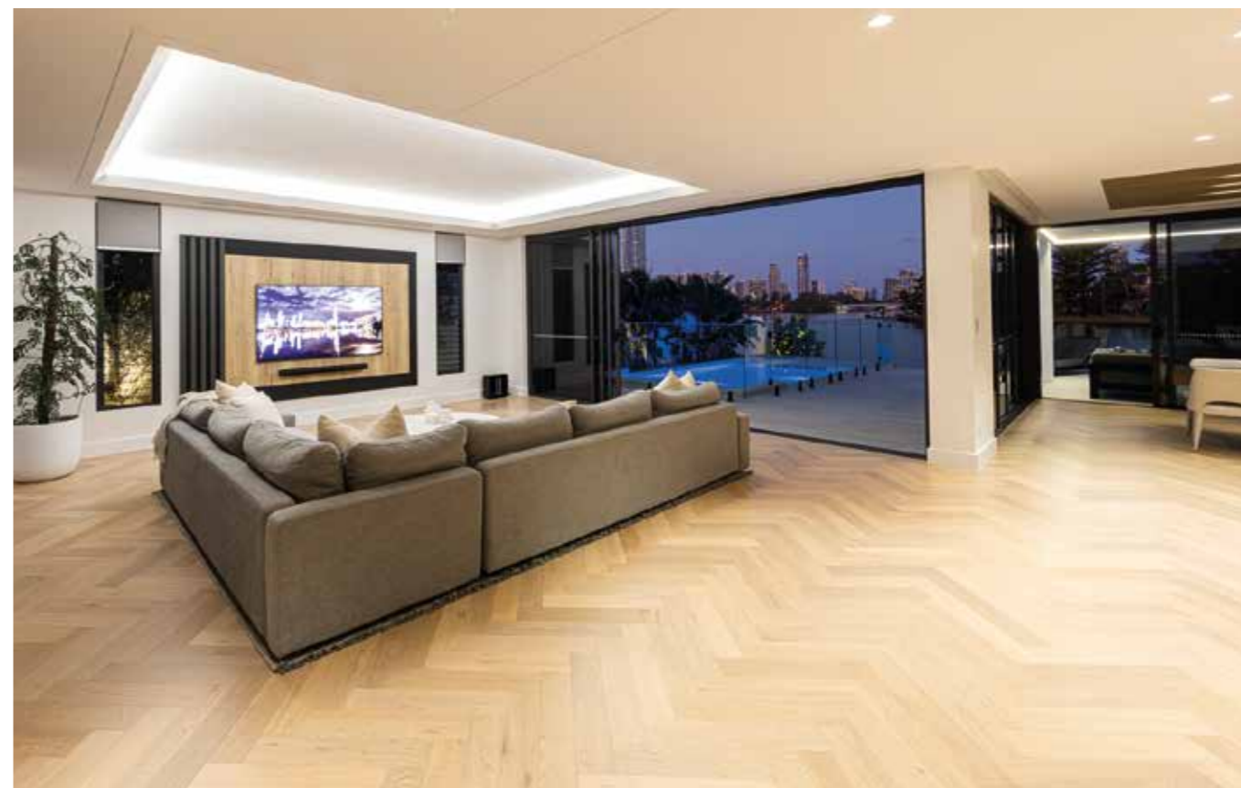
ABOVE. Wood floors were installed in a herringbone pattern in several environments of the ground floors with ULTRABOND ECO S955 1K after preparing the substrates with ECO PRIM T PLUS and ULTRAPLAN ECO.
