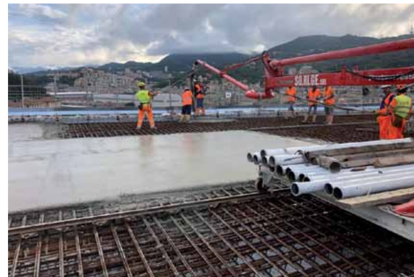
DYNAMON XTEND W202 N, DYNAMON LZ 551 and EXPANCRETE PLUS admixtures were supplied for the concrete poured on the deck.
