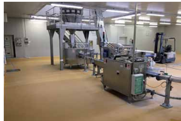
Vegetables processing plant – MAPEFLOOR CPU/NZ.
