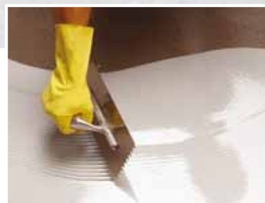
Application with Mapefloor CPU
