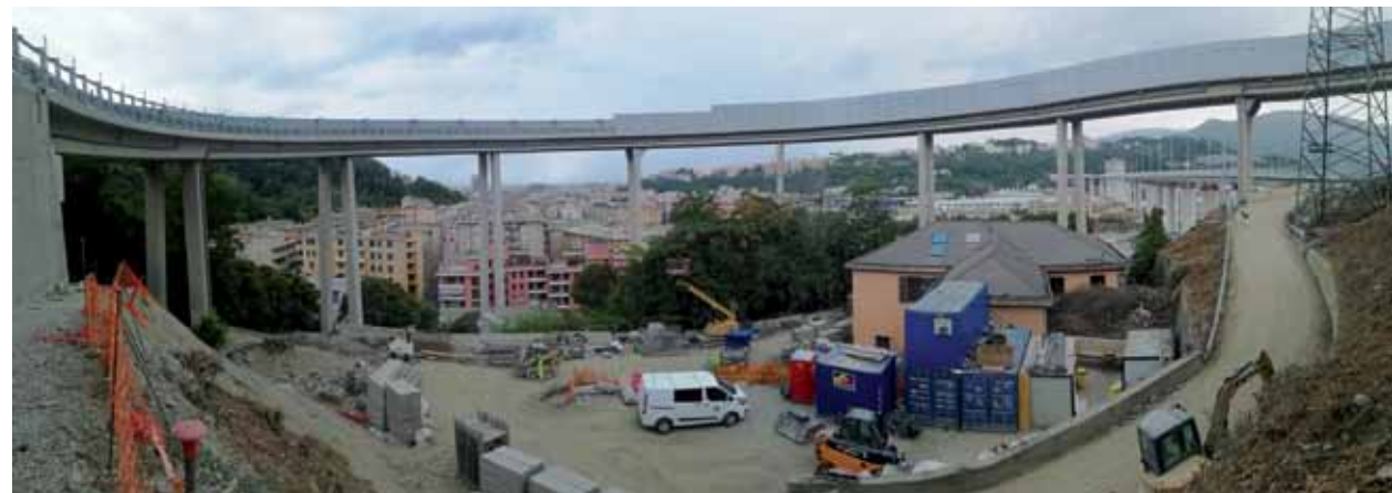
ABOVE. Repair work was carried out on both the intrados and the extrados of the bridge deck. Various products by Mapei were used for the job, including MAPEGROUT EASY FLOW fibre-reinforced thixotropic mortar and the hi-flow mortars MAPEGROUT GF BETONCINO B1 and MAPEGROUT HI-FLOW B2.
