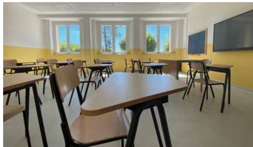
Apart from the structural work, the project also included a completely new look for the classrooms by applying cementitious floorings made with the ULTRATOP LOFT system.
