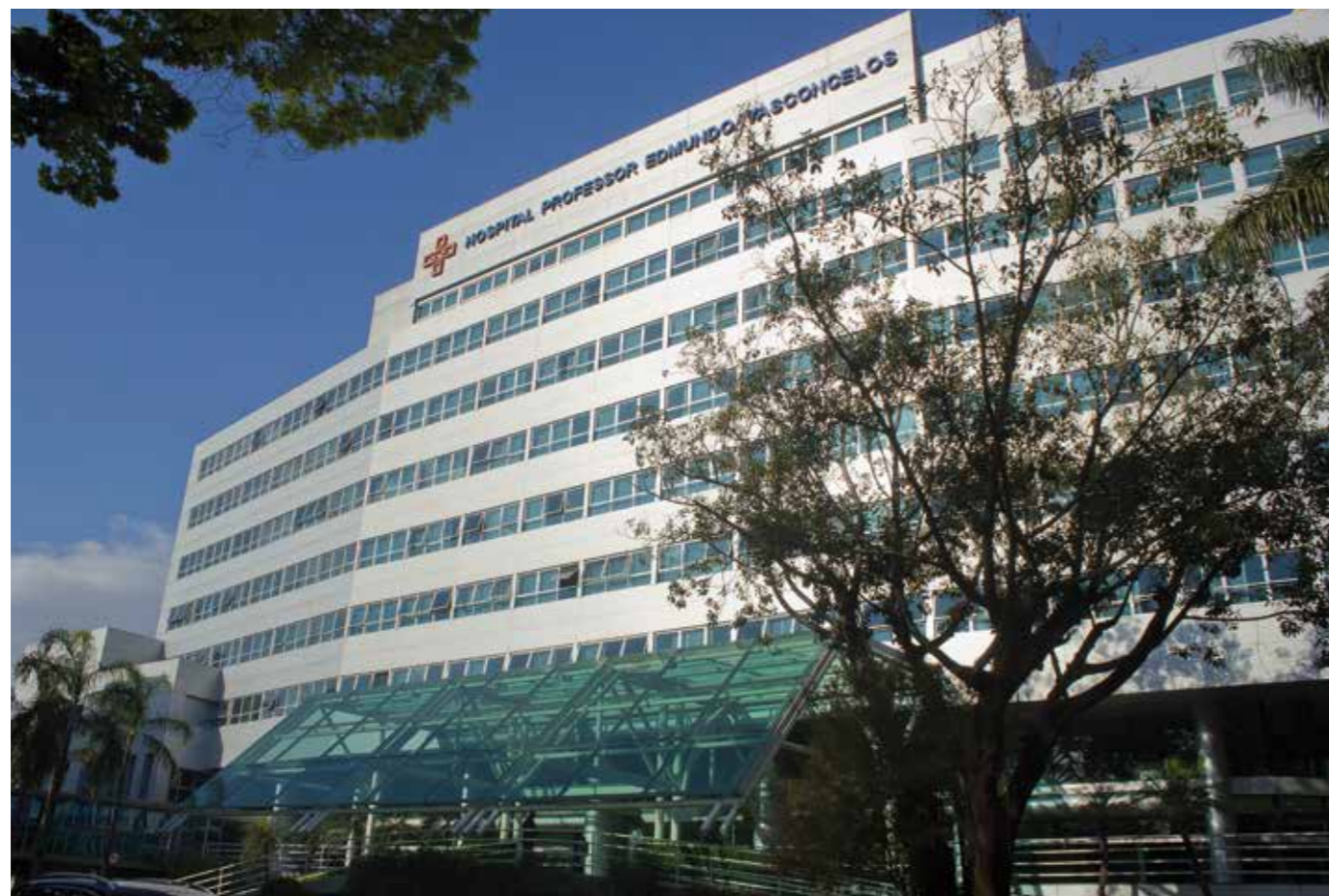
ABOVE. Edmundo Vasconcelos Hospital was originally designed by Oscar Niemeyer and renovated in 2017-2018. TOP THE PAGES. Sheet vinyl floorings by Gerflor were bonded with MAPECRYL ECO adhesive in the corridors, waiting and communal areas, after preparing substrates with TOPCEM and ULTRAPLAN ECO.
